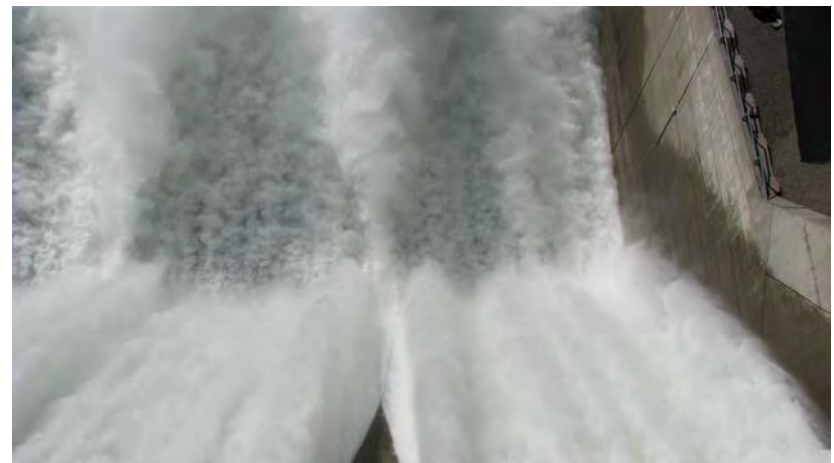
B. Spill jet transition during 7 kcfs/bay
