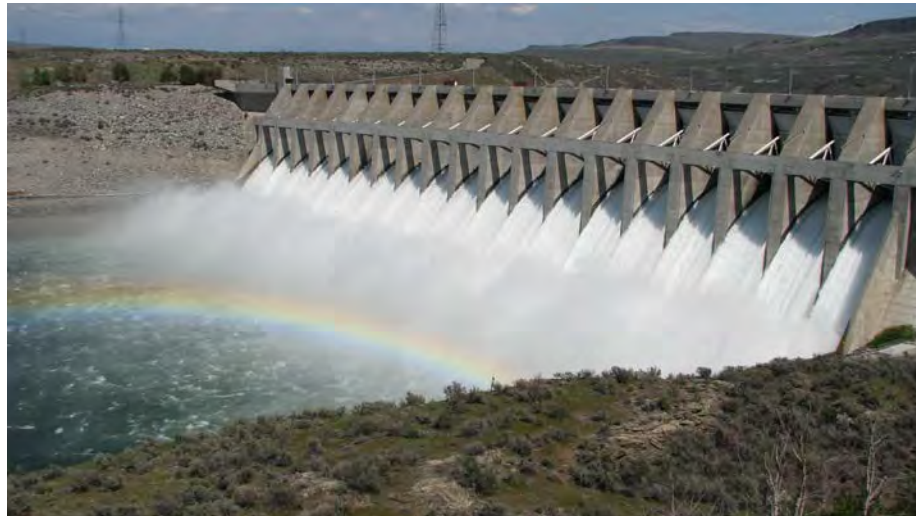
B. Aerated Spillway Flow during 58 kcfs event.
