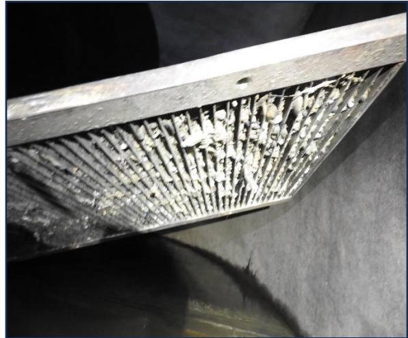
JBS makeup water valve grate underside
