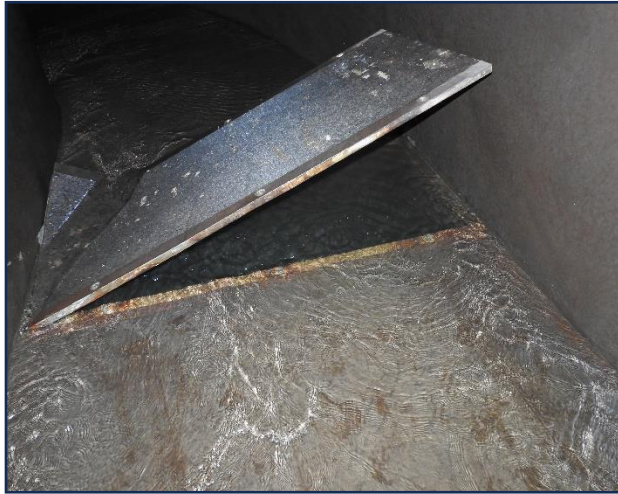
JBS makeup water valve damaged grate cover
