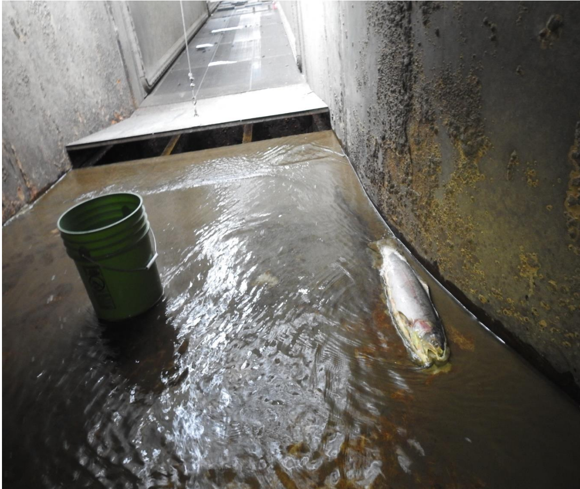
JBS channel to emergency bypass release pipe; fish mortality location
